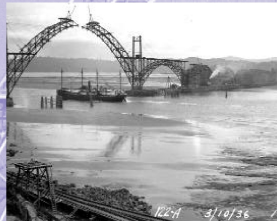
Yaquina Bay Bridge in Oregon, above and background, 1936. The bridge was metalized in 1992. Courtesy of the Oregon DOT
