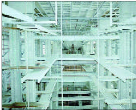
Interior scaffolding for metalizing Courtesy of Great Western Corporation
