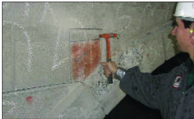
Sounding for delaminated concrete Courtesy of Great Western Corporation
