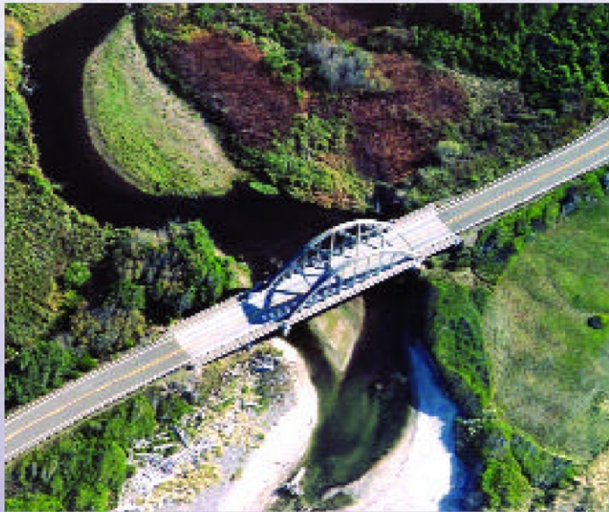
Big Creek Bridge in Oregon, another completed metalizing-cathodic protection project. Courtesy of the Oregon DOT
