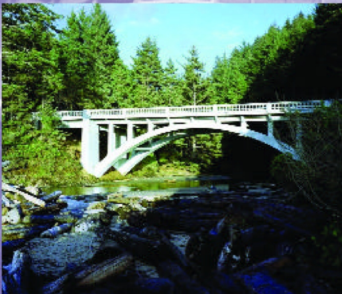
Cummins Creek Bridge in Oregon, a completed metalizing-cathodic protection project. Courtesy of the Oregon DOT
