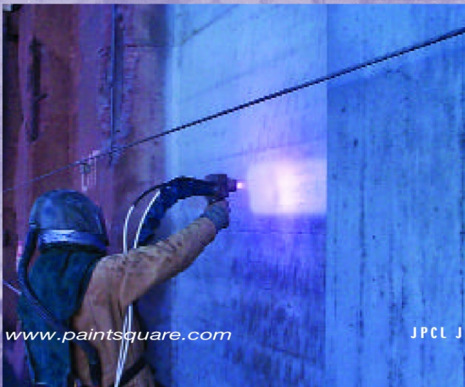
Metalizing concrete surface Courtesy of Corrosion Restoration Technologies
